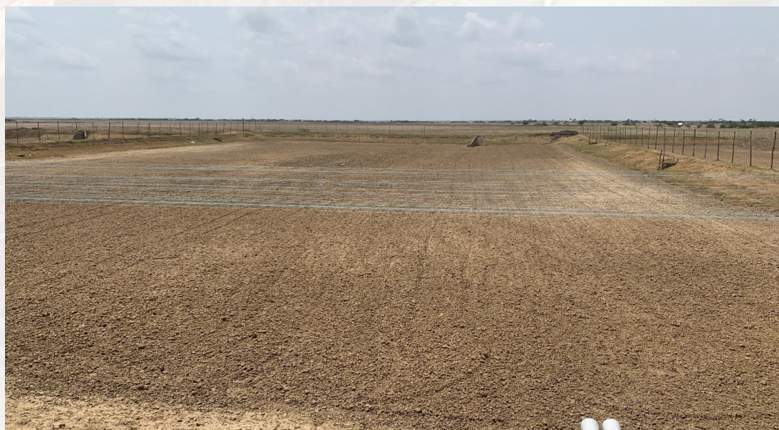
Figure 1: Thoroughly prepared pond bottom before filling in water
