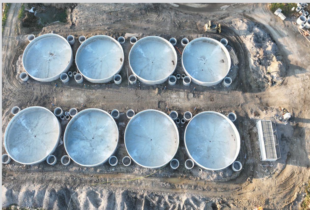
Figure 3: An aerial view of a newly constructed Tank-By-Pond (TBP) System where each tank is equipped with four airlift column aerators and a swirl separator
