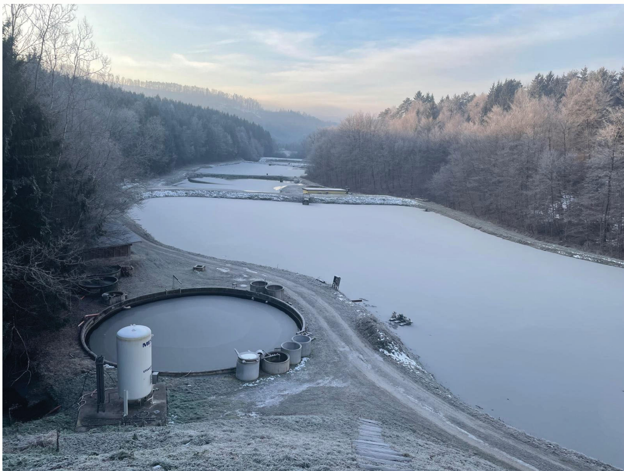
Figure 1: TBP system with 15 m diameter tank (Fish farm Žabnik (Slovenia), G2O d.o.o.)
